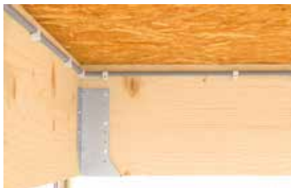
Cable fixing
