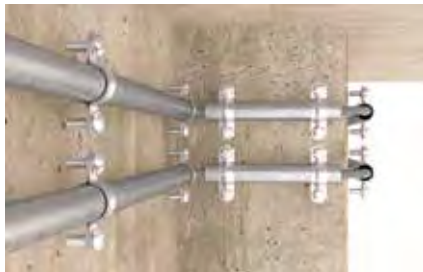
Fixing steel armoured conduits
